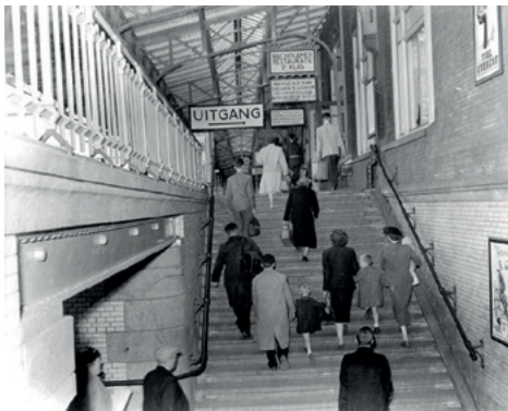
De personentunnel in 1954 (HUA)
